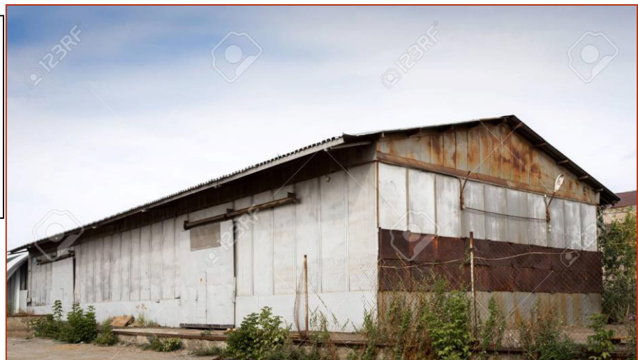
Picture 2: Old brown warehouse with sheet metal cladding with street lights.
